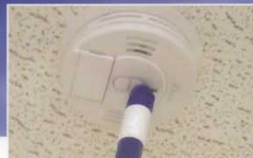
Test your smoke alarm once a month with the end of a broom handle
